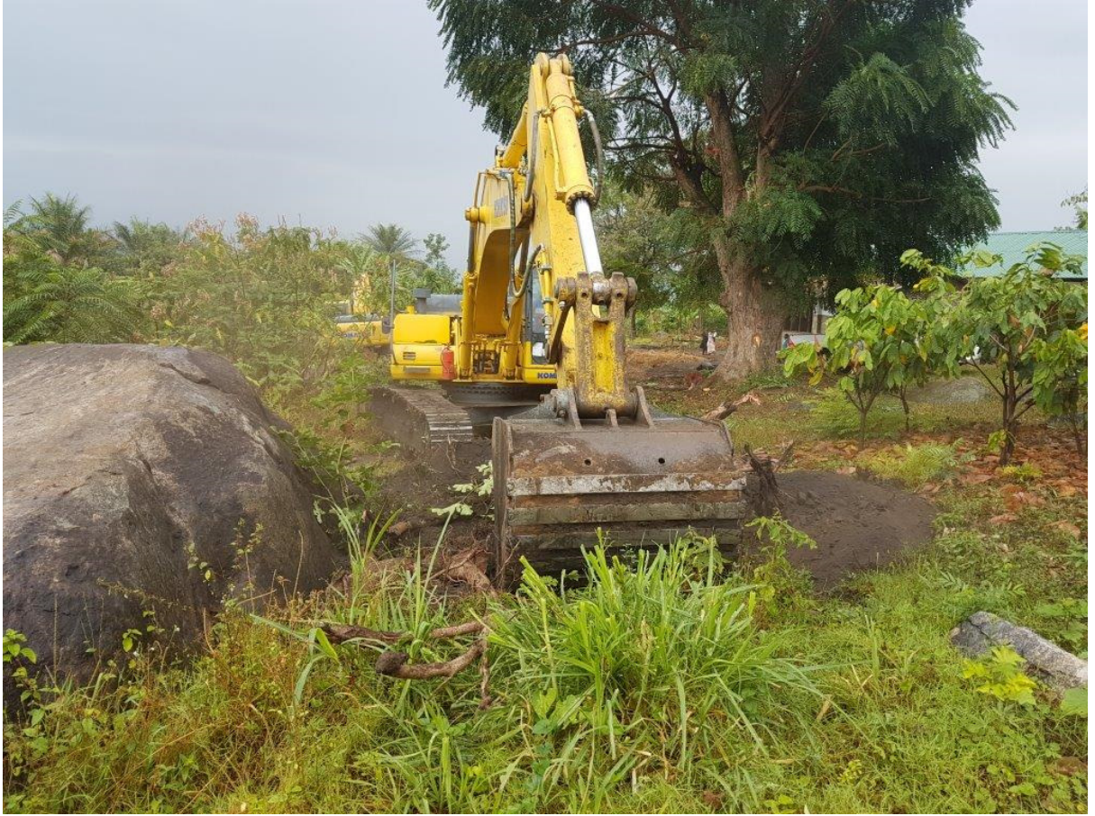
Ground clearing for the Sindila hydropower project powerhouse
